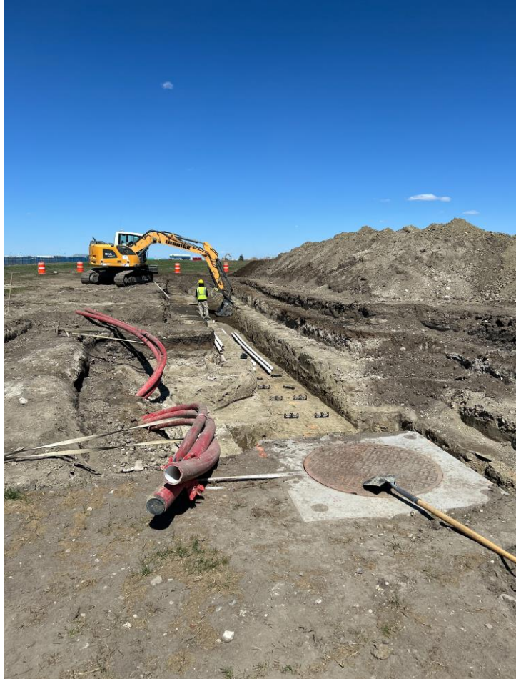
Duct Bank Installation
