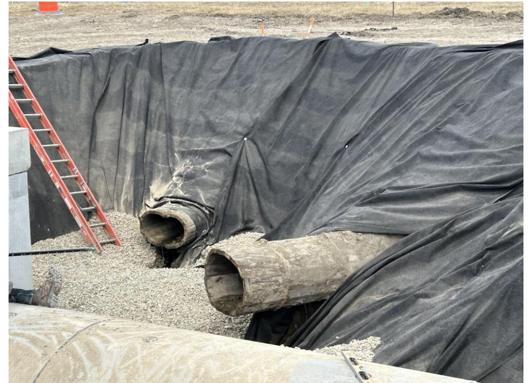
Storm Line Installation & Wooden Pipe Replacement
